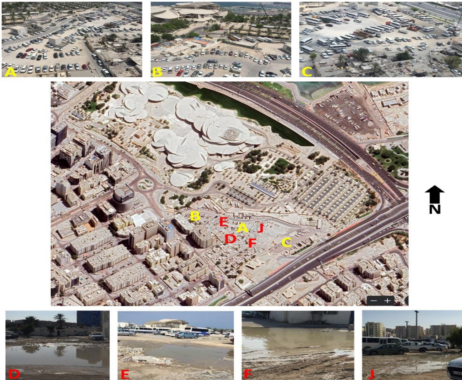
Figure -17: The effect of rainwater on neglected lands that are used as random parking lots. (Source: The
